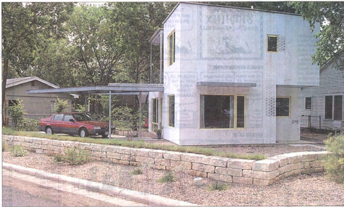
The second-story porch and the large windows on both floors all look north to Bruning Avenue. The windows bring natural light inside and connect the rooms to the street outside. A low retaining wall and a short berm of buffalo grass provide a physical barrier to the street without isolating the house from the neighborhood outside.
