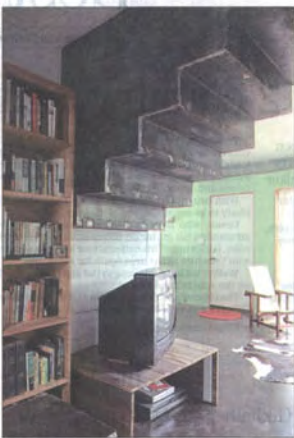
In architects Cindy and Rick Black's 980-square-foot home, the underside of the steel staircase separates the study/guestroom from the living room. Shiplap walls reflect the flavor of the older homes in the neighborhood.
